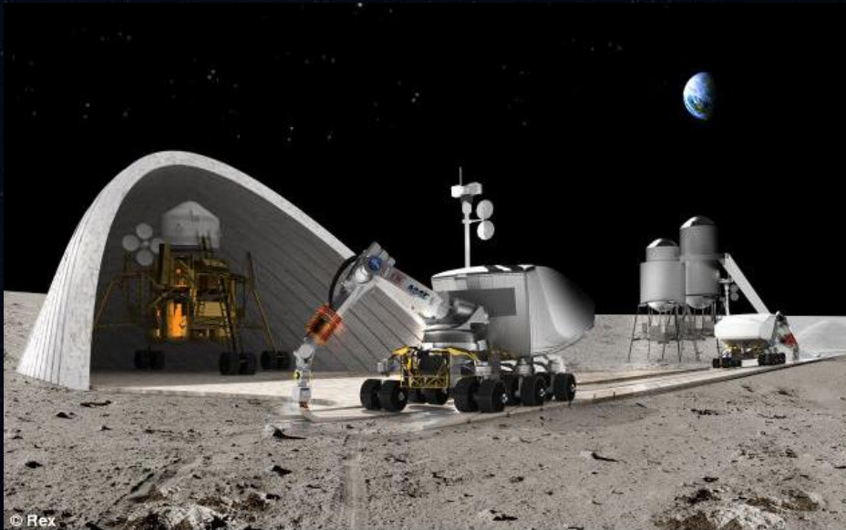
Concept for a lunar base built by construction robots and a form of 3D printing known as contour-crafting. Credit: NASA
